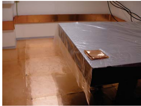
(b) Interior view during construction 1. The central ground plane for the room is a copper band attached to the wall.
