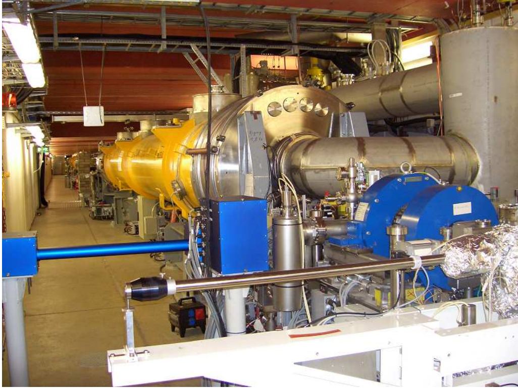
Figure 1.2: FLASH accelerator tunnel (self-made photo).
