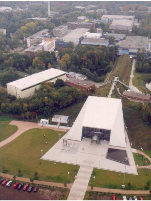
Figure 8: Photograph of TTF2 at DESY. The hall in the background is housing TTF1, and in the foreground the experimental hall for scientific users of TTF2 FEL is seen.
