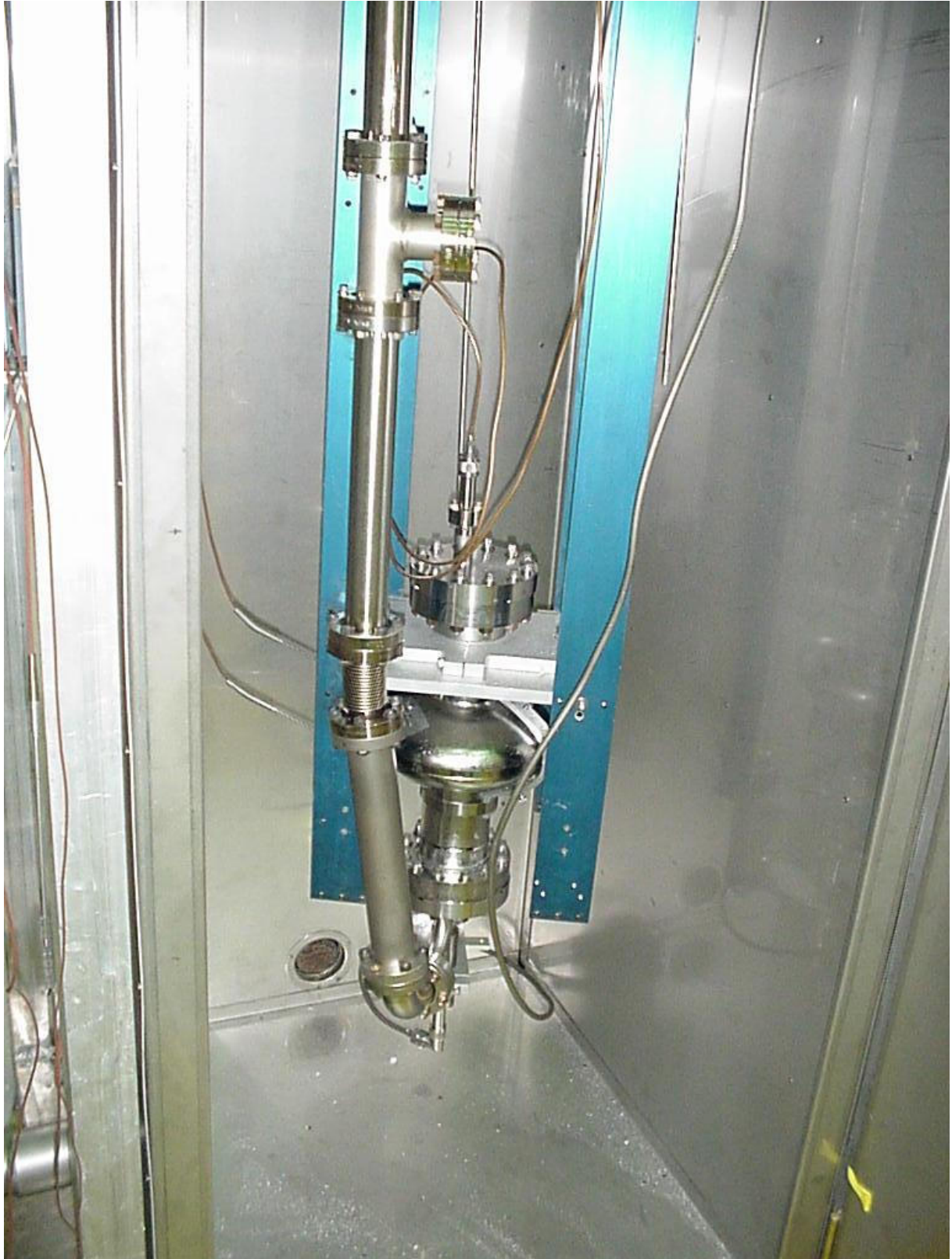
Figure 15: Installation at Jefferson Lab for “in-situ” baking.
